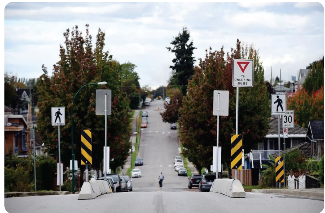
Adanac Overpass in 2018.
