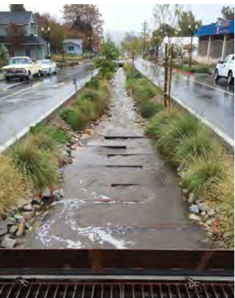
Bioswale (The City of Paso Robles)
