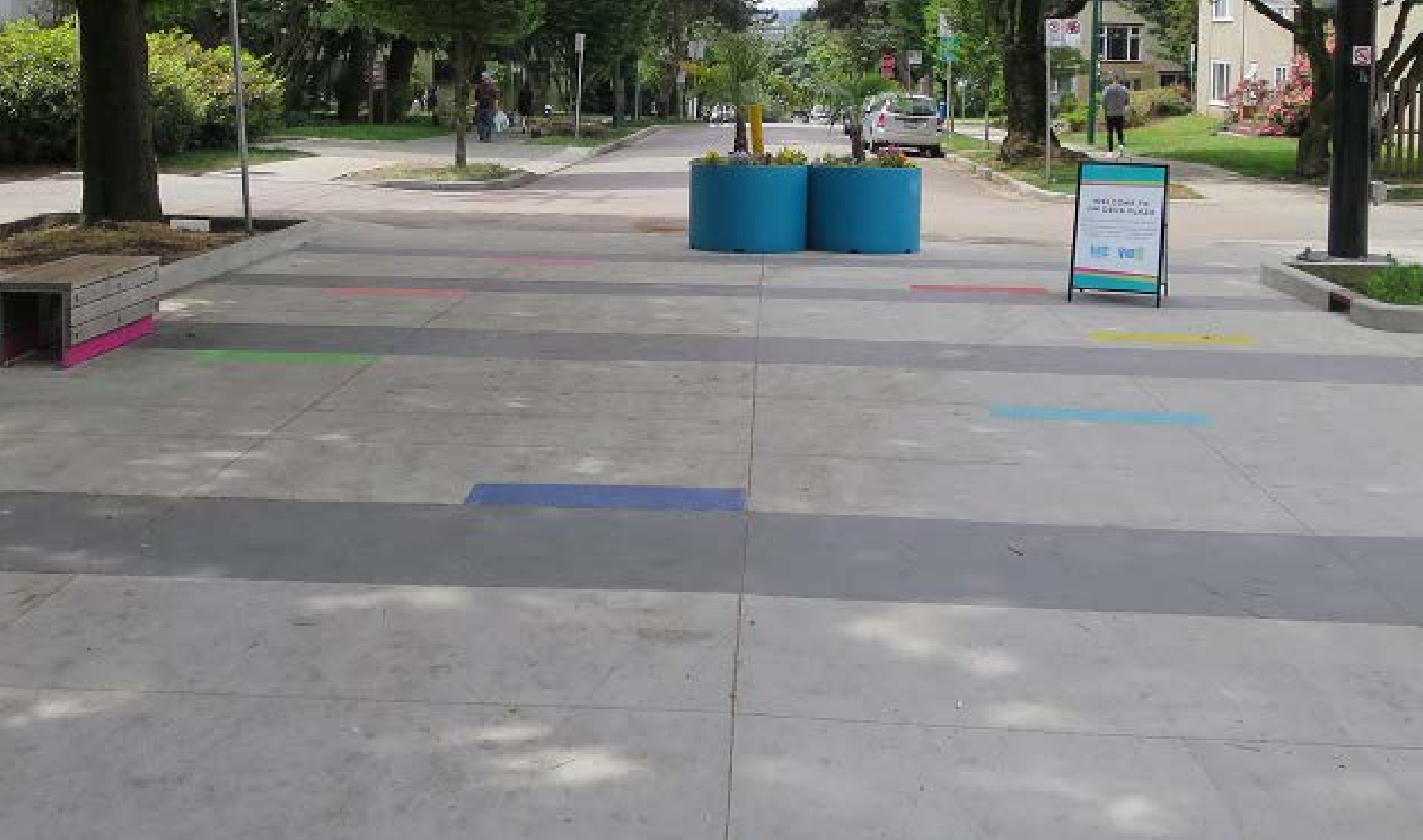
Continuous concrete paving pattern between Haro and Robson streets.
