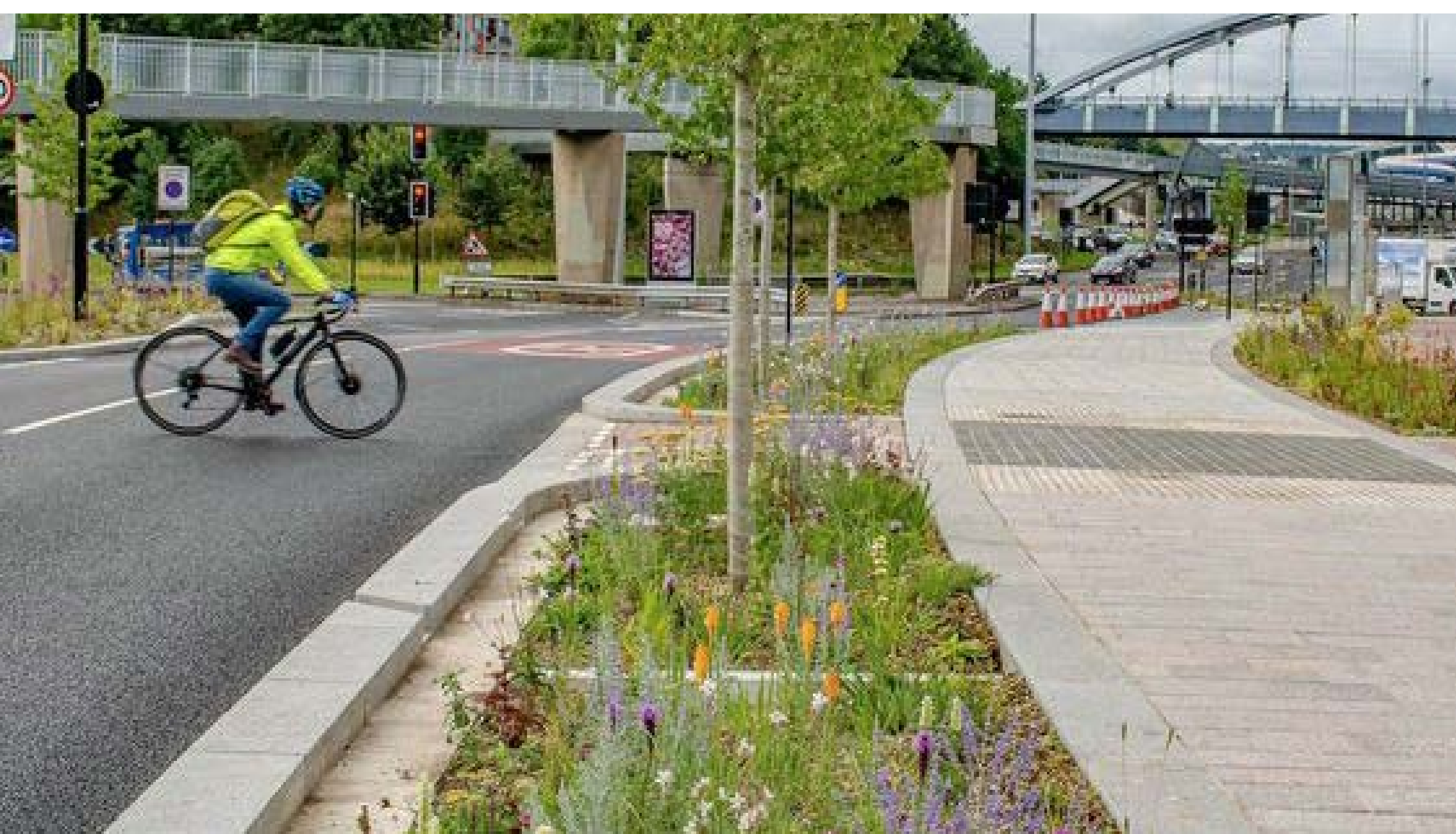
Green rainwater infrastructure elements such as rain gardens, planting and tree trenches to manage urban rainwater runoff.
