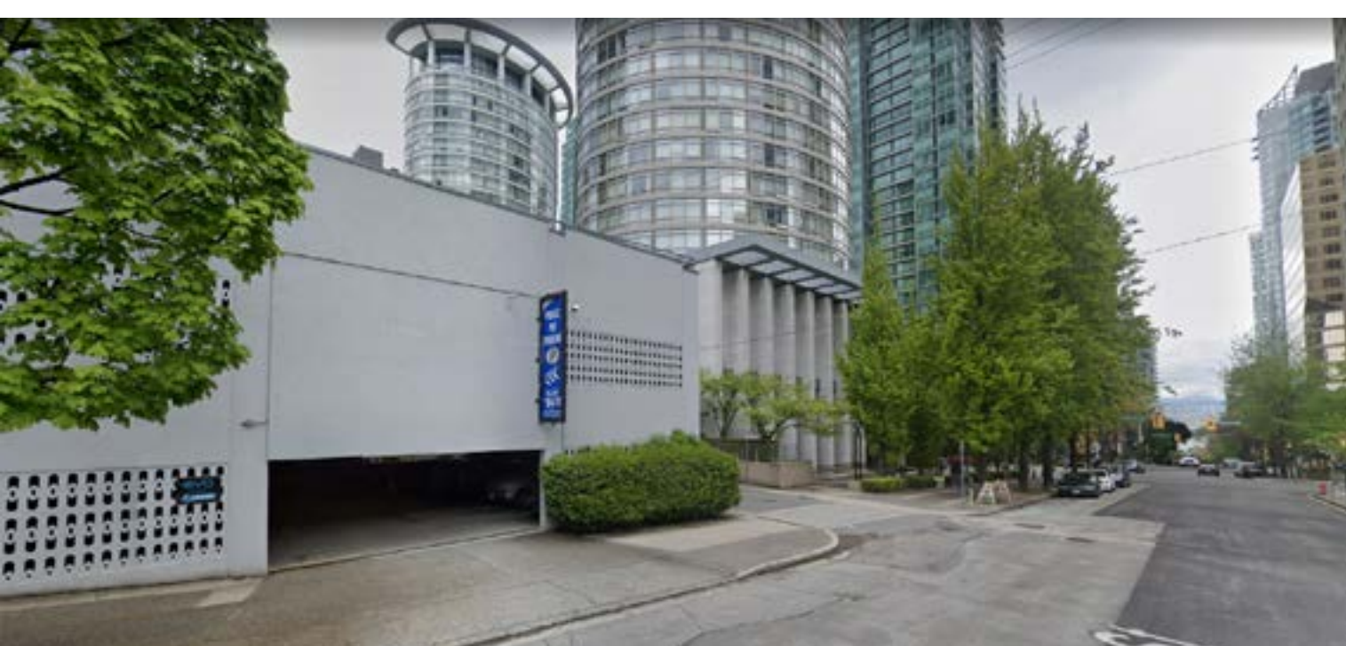
Retained access to parkade
