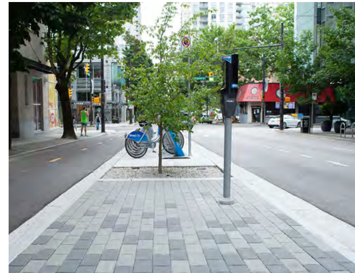
Permeable pavement with rainwater tree trenches (Richards Street, Vancouver)
