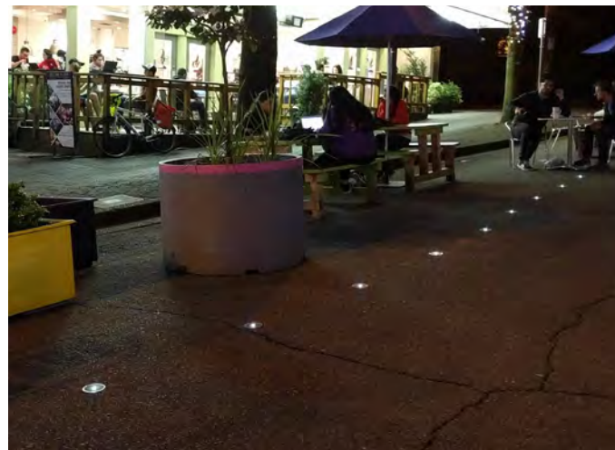
Solar in-ground lights
