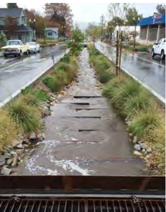
Bioswale (The City of Paso Robles)
