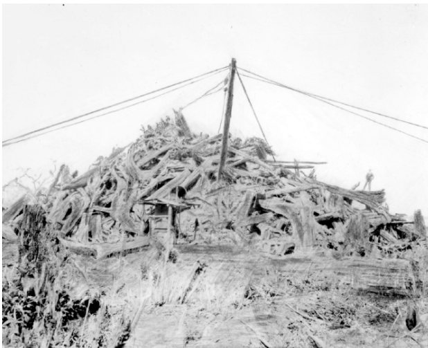
Figure 93. Clearing timber Quilchena 1926
