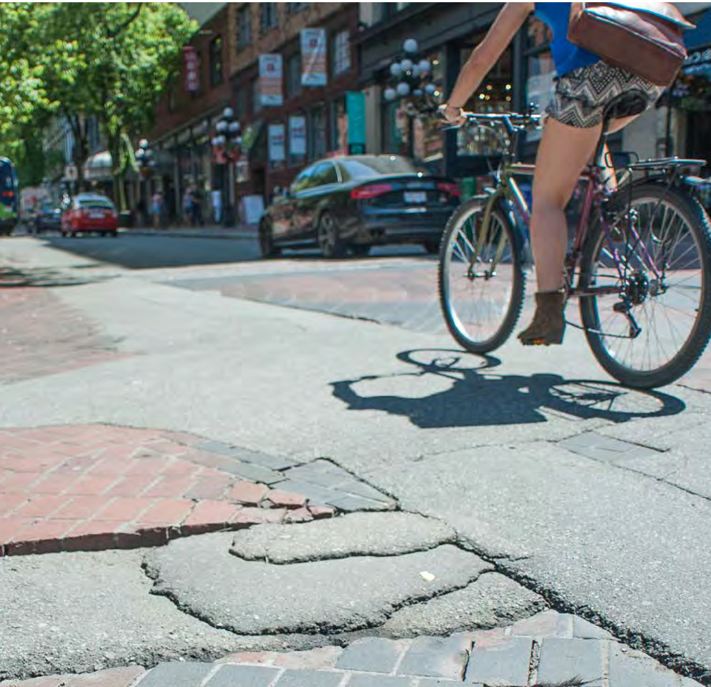
The deteriorated pavers result in safety hazards and accessibility obstacles for pedestrians, especially those using strollers or mobility devices.
