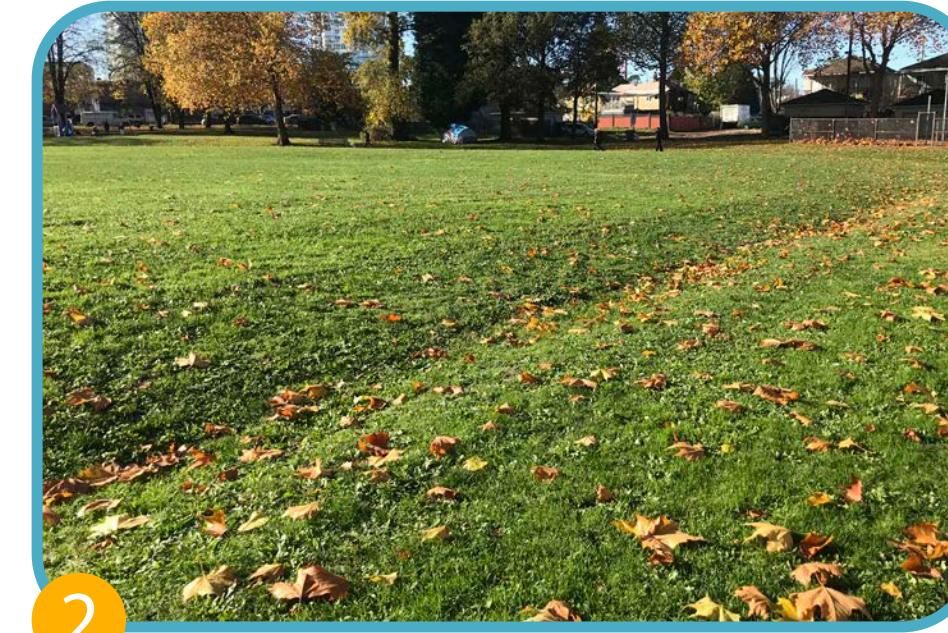
2 Grass field Low points along the edge of the field for drainage creates a trip hazard for users of the sports field
