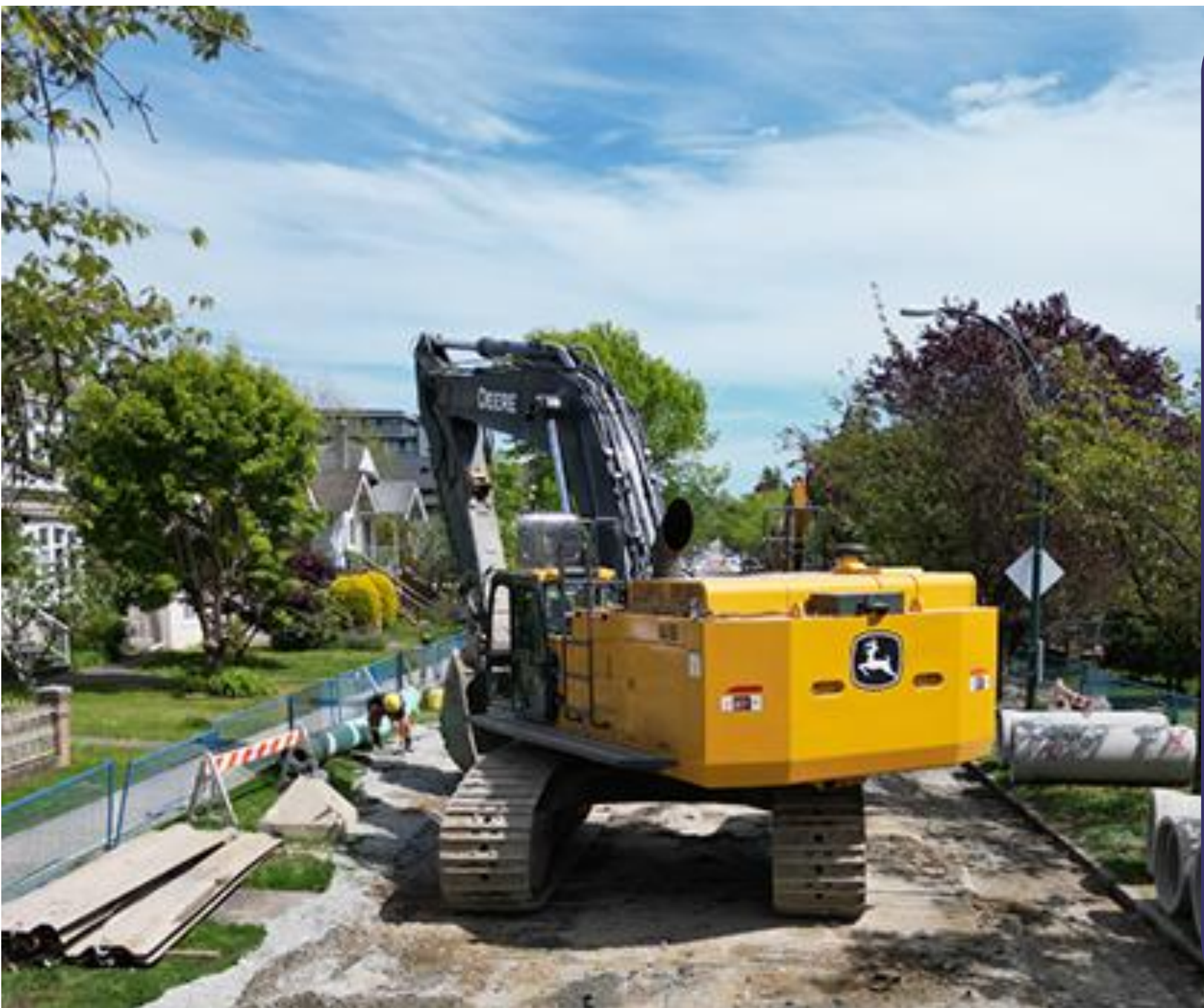
Excavator working on sewer separation at West 49th Source: City of Vancouver
