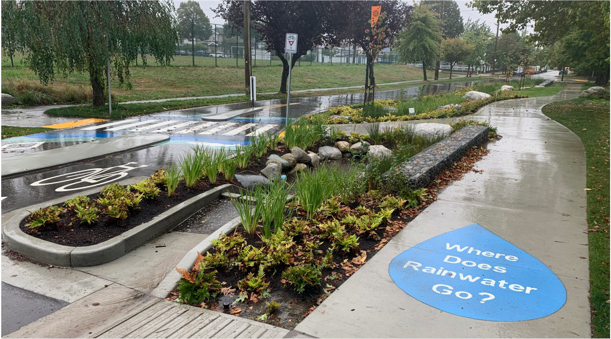
Green rainwater infrastructure like rain gardens and tree trenches to manage rainwater runoff.
